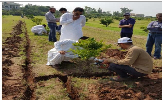
Trenching for Orchard Demonstration Plot
