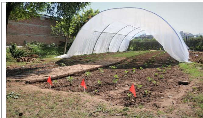
Installation and Laying of GrowStream Pipe in Vegetable Demonstration Plot
