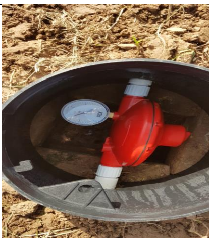
Automatic pressure regulator (APR)- mechanical device
